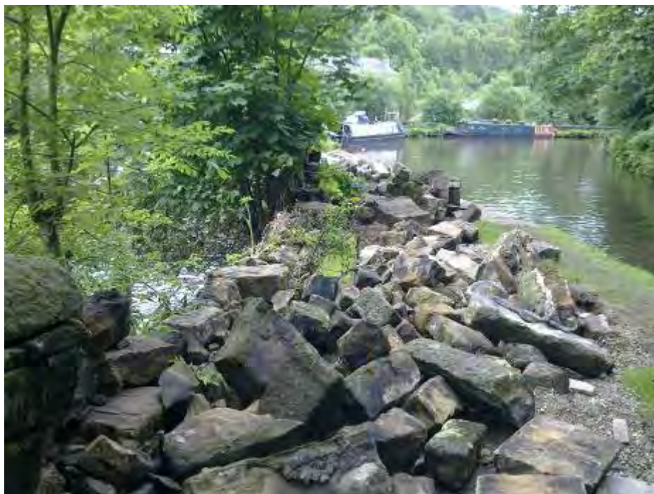
Figure 8: River Calder river wall breached and flowed into canal (Source: EA & CRT)
