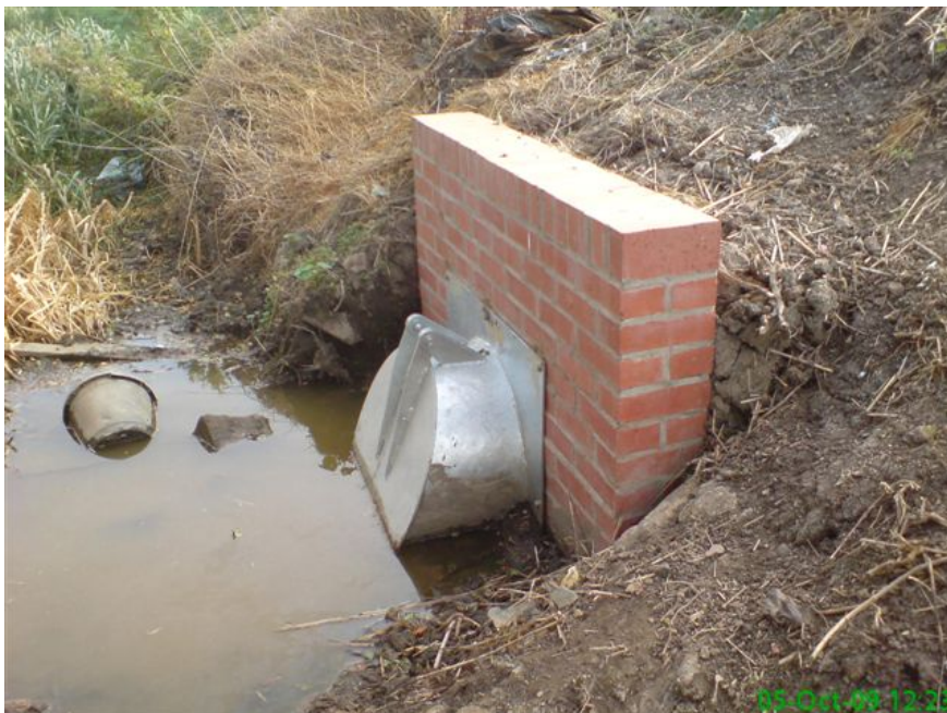
Figure 18 : Flap valve installation at the northern end of Hook Drain
