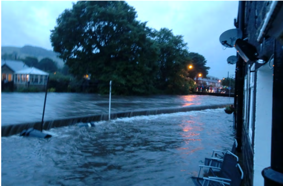
Figure 12 - Flood waters overtopping river wall downstream of Caldene Bridge (Source: CMBC).
