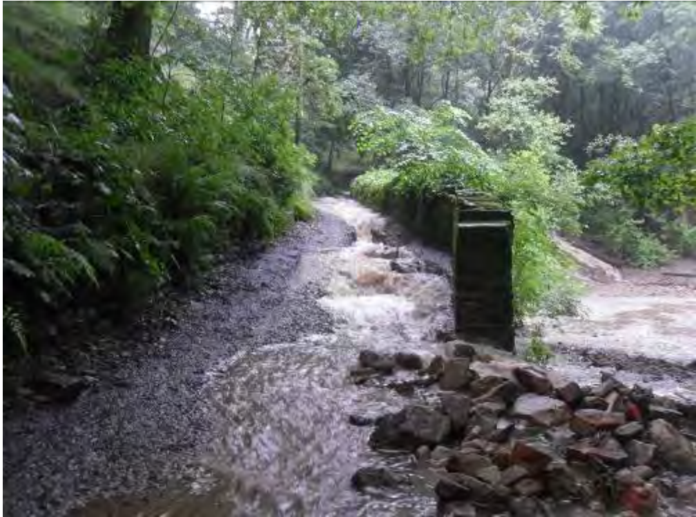
Figure 2 - The access track adjacent to Nutclough Reservoir being eroded by floodwaters from the spillway, which flowed onto the A6033.
