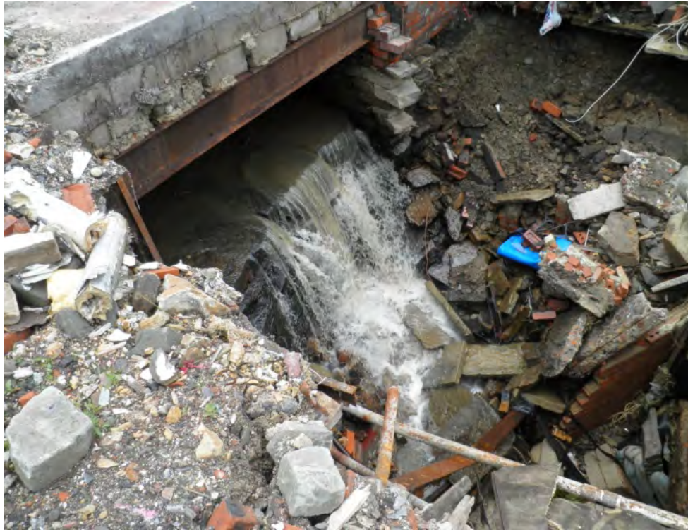
Figure 3 – The collapsed culvert on Red Water Clough, Cornholme (Source: EA)
