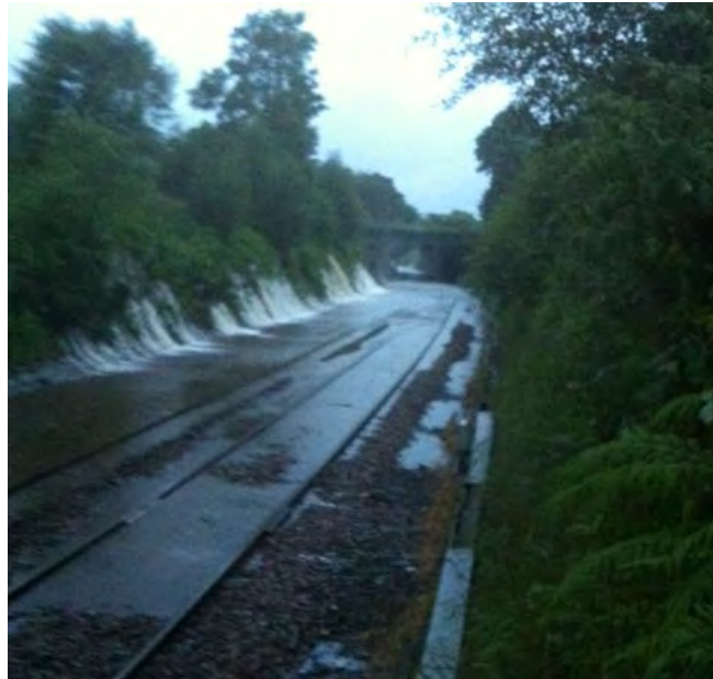
Figure 4 – Flood waters spilling onto the rail track downstream of Dean Royd Road (Source: Network Rail)
