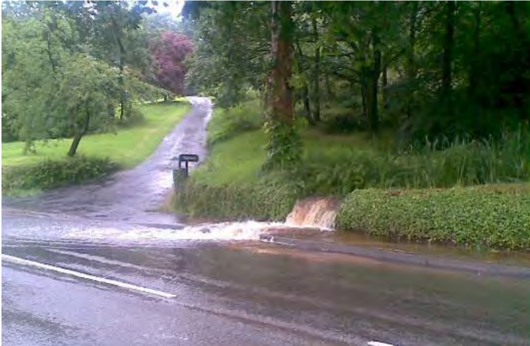
Figure 11 - A typical example of a watercourse in Cragg Vale bypassing the drainage system flooding the highway.
