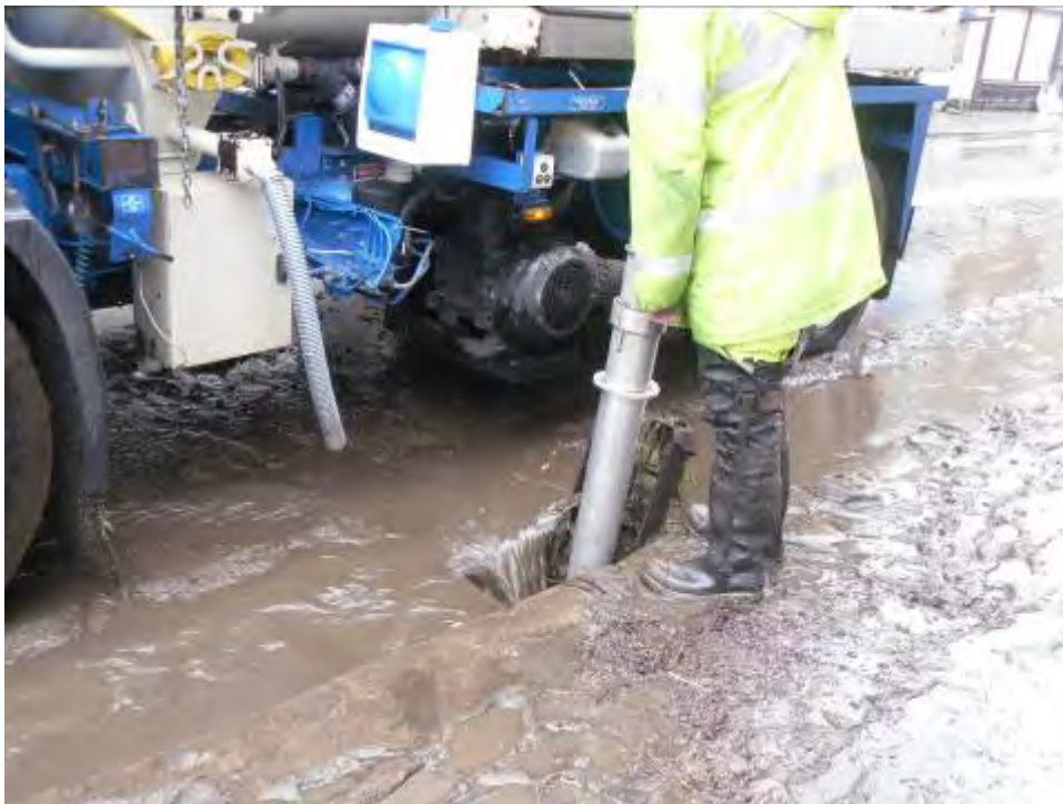
Figure 12 - Drainage contractor unblocking the highway drains in Hebden Bridge.
