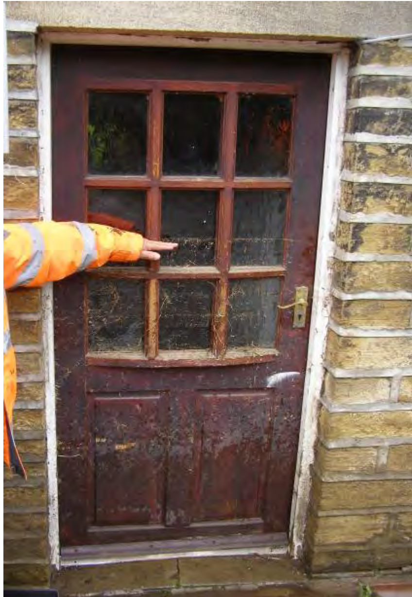
Figure 12 – The rack mark on the property door shows the height the flood waters reached at the peak of the rainfall event.
