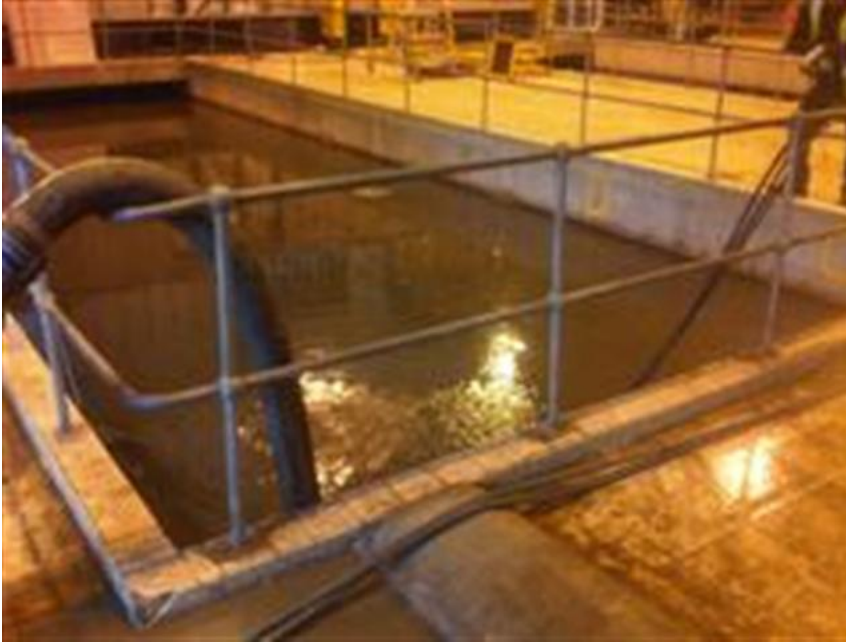
Figure 11 : Dry Well at Carr Lane PS flooded
