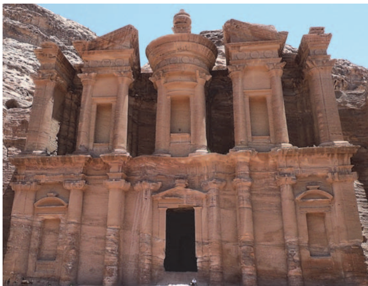
FIGURE 1 The Monastery at Petra, Jordan, capital city of the Nabataean kingdom (ca. 300 BC). This heritage site, carved out of a sandstone cliff, shows extensive damage due to salt weathering. Note the salt efflorescence (mainly halite) on the bottom part of the structure, shown by extensive white areas, and the loss of relief of carved elements such as the columns. Saline solutions rising from the ground evaporate at the surface and subsurface of the porous stone, thus resulting in salt efflorescence and deleterious sub-efflorescence. Daily and seasonal temperature and humidity changes also result in damage due to cyclic salt dissolution–crystallization events. Treatment of the sandstone with crystallization additives such as ferrocyanide could help prevent salt damage. PHOTO: M. GÓMEZ HERAS
