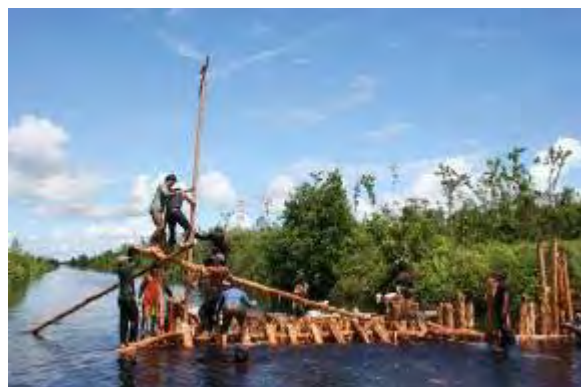
Figure 9.4: Peatland restoration. Blocking of a canal in degraded peat swamp forests in Central Kalimantan, by local communities using manual traditional techniques (photo: Marcel Silvius, Wetlands International).
