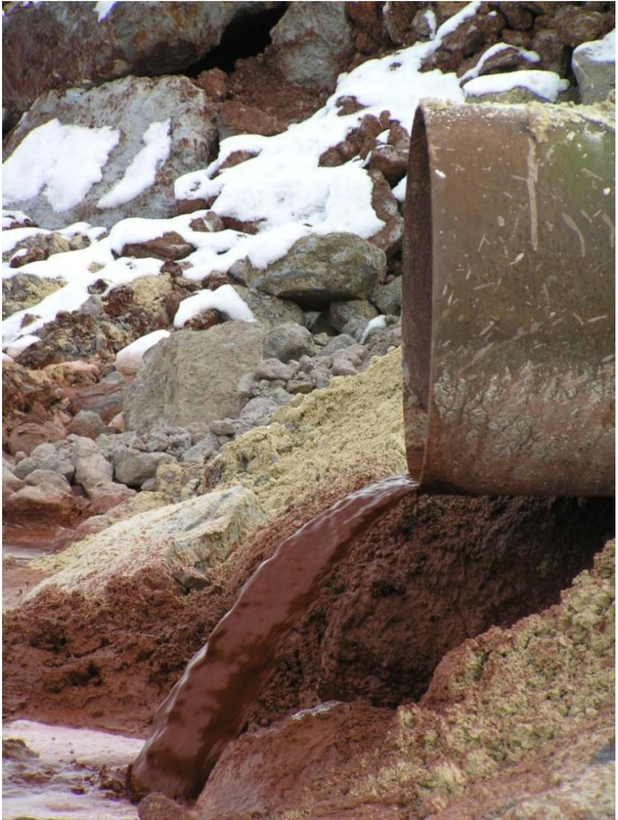
Figure 1. Red mud slurry continued drained from the breached Ajka dam (into rapidly constructed containment lagoons) for several weeks after the spill.
